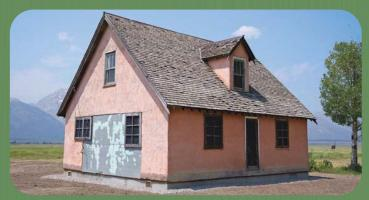
The Pink House sits on its new foundation, which will eliminate further damage to the building's structural integrity and stucco siding.
