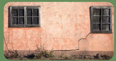
The Pink House's stucco was severely cracked due to the building's failing foundation and decades of exposure to the elements.
